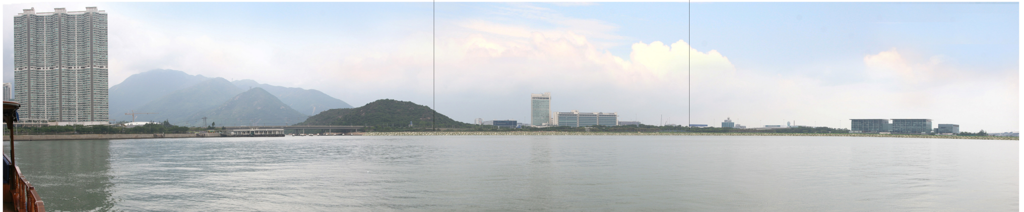
Development without Mitigation (Construction Phase)
