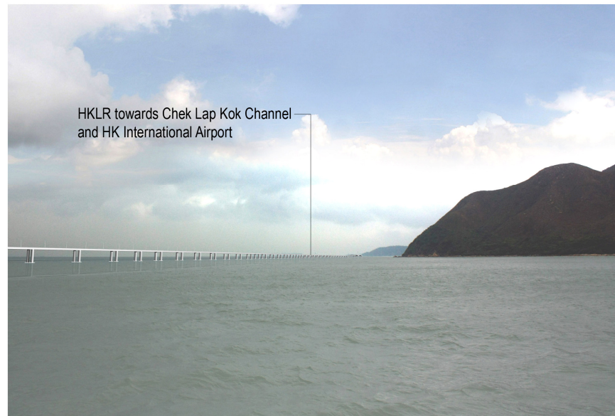
Development without Mitigation (Construction Phase)
