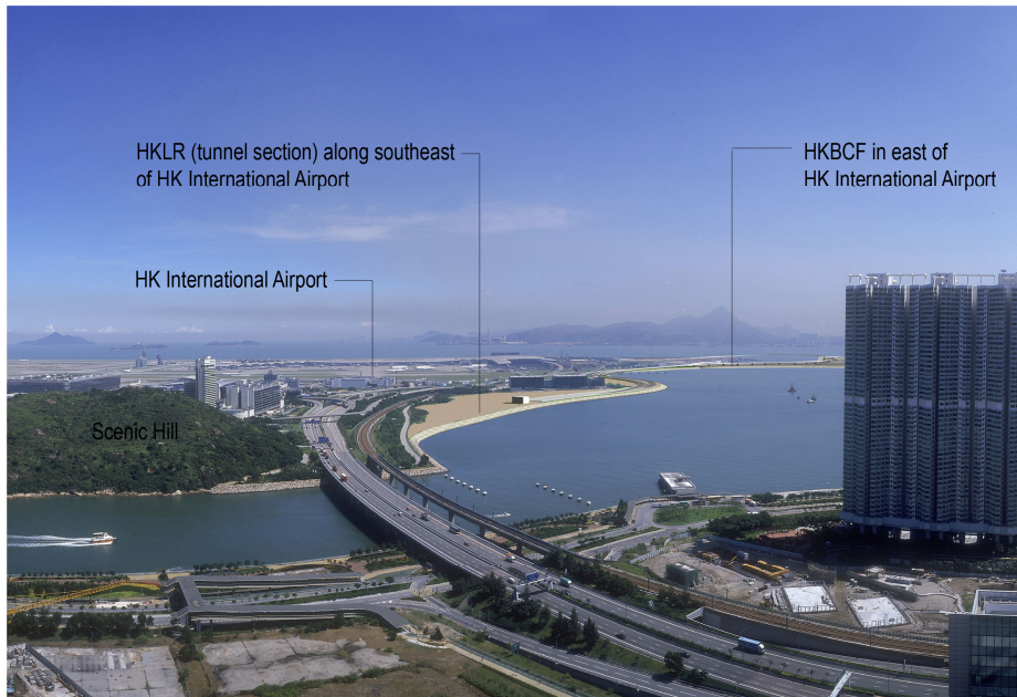
Development without Mitigation (Construction Phase)
