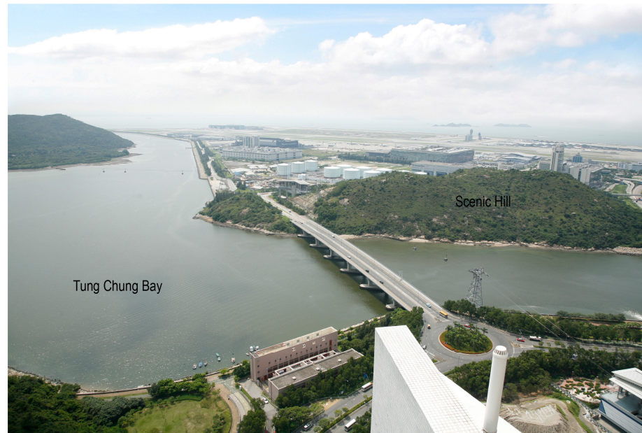
Existing Baseline Condition
