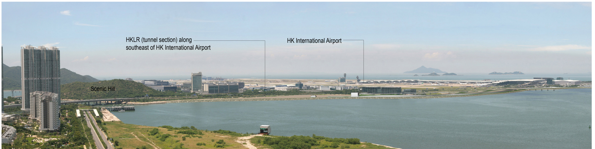
Development without Mitigation (Construction Phase)
