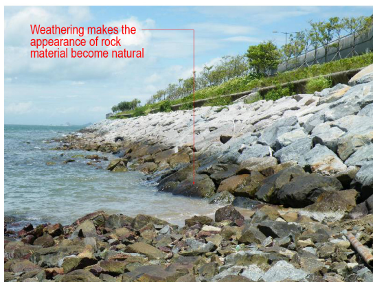
Example of 'Natural-look' Artificial Seawall
