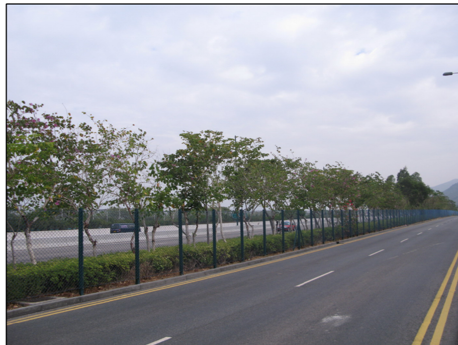
PHOTO A17 - LR10 ROADSIDE PLANTING ALONG NORTH LANTAU HIGHWAY AND WITHIN MTR SIU HO WAN DEPOT
