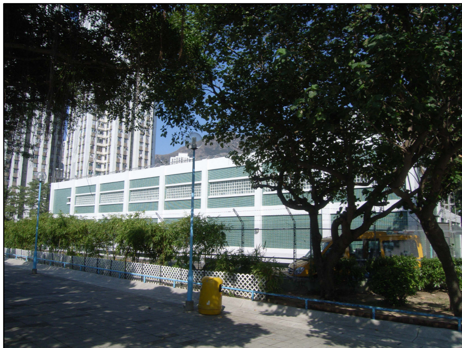
PHOTO C01 - GIC1 WORKERS OF SALT WATER PUMPING STATION NEAR MEI LOK LANE
