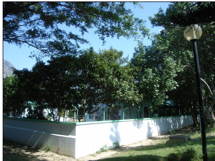
PHOTO C02 - GIC2 WORKERS OF PAK KOK SEWERAGE PUMPING STATION
