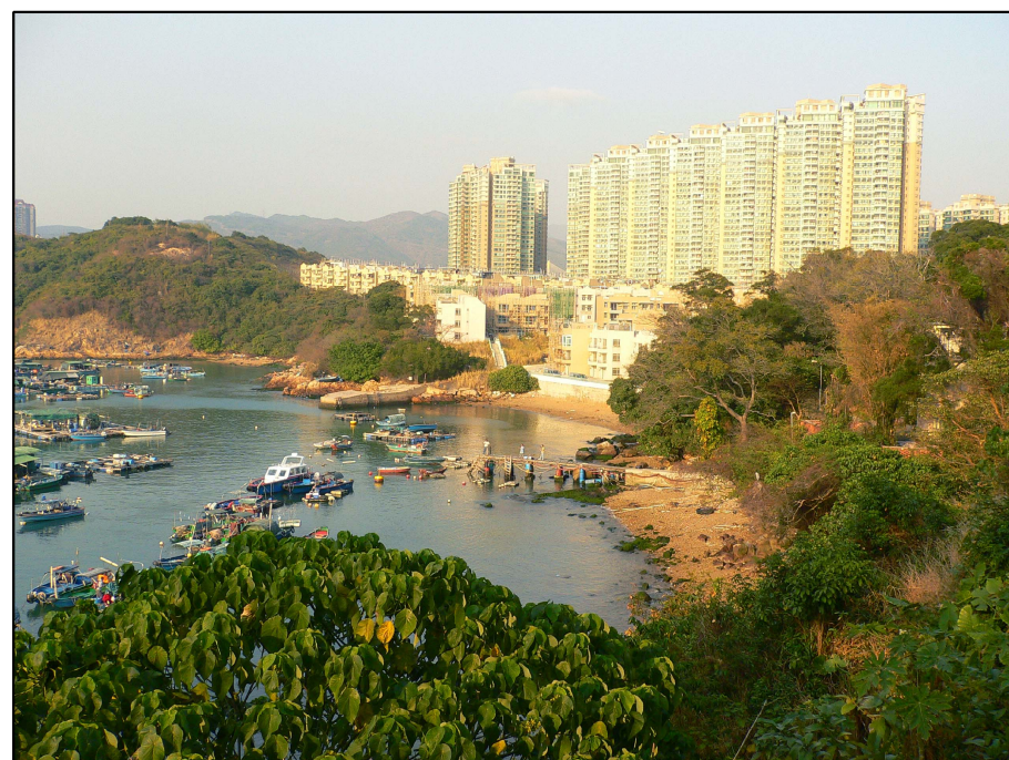
PHOTO E05 - D3 MA WAN RESIDENTIAL AREA
