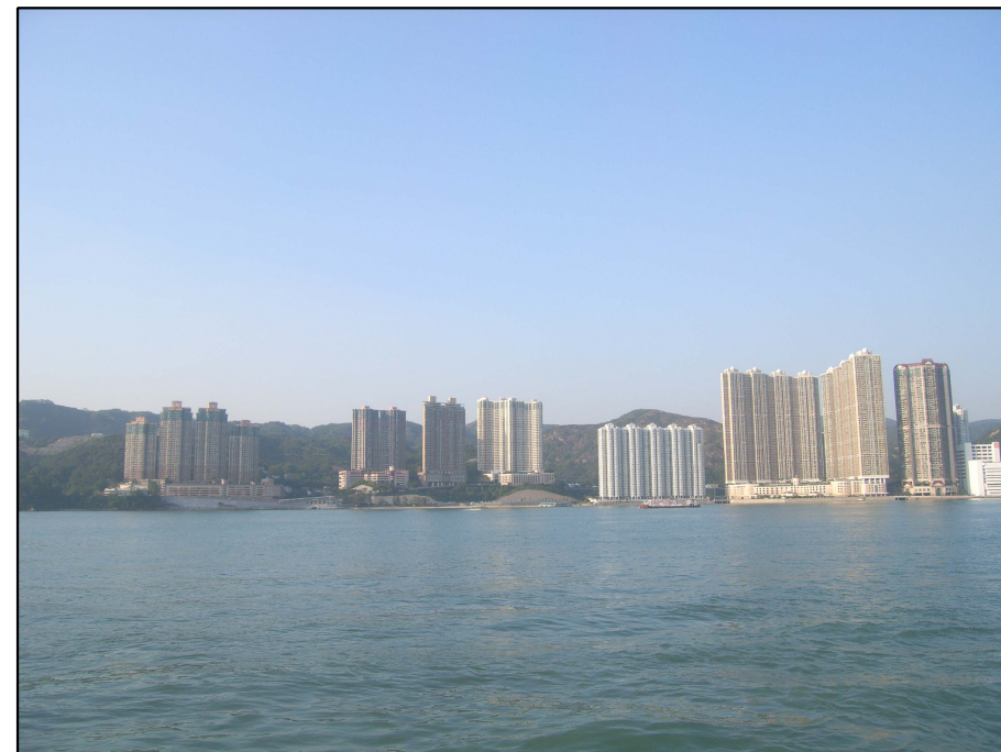
PHOTO E03 - D2 TSING LUNG TAU, SHAM TSENG AND TING KAU RESIDENTIAL AREA
