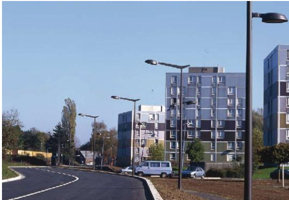
Possible example of highways lighting
