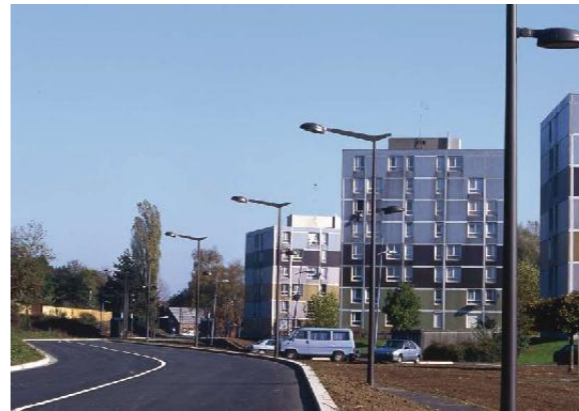
Possible example of highways lighting
