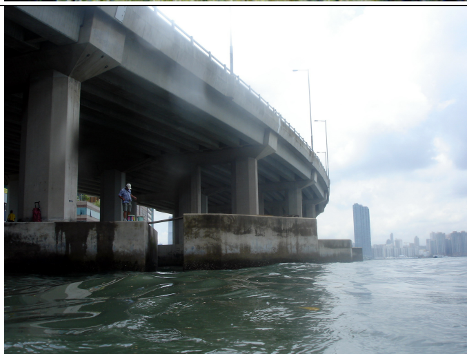
Plate 18. The eastern Corridor structure.
