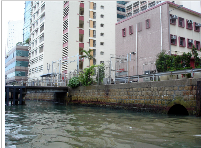
Plate 13. The seawall at the North Point Landing Point.
