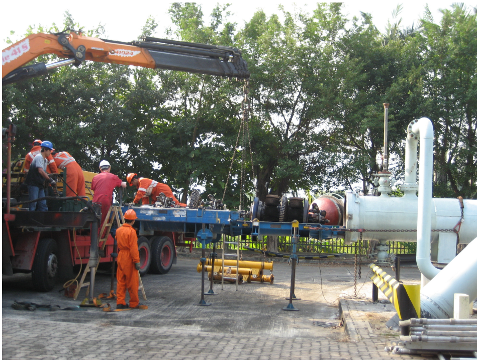
Photo: Installation of the pig during pigging operation
