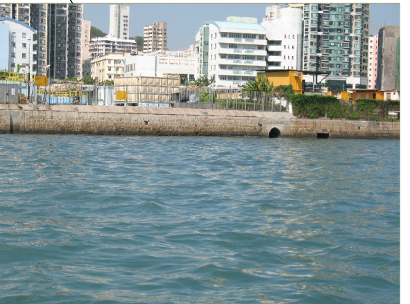
VERTICLE ARTIFICIAL SEAWALL ALONG THE SHORE OF MA TAU KOK
