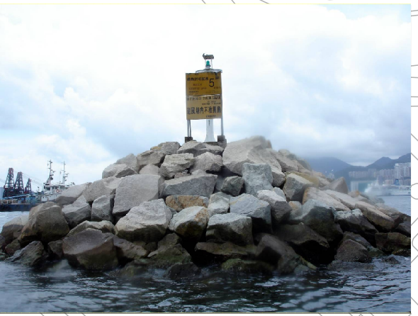
BREAKWATER MADE OF ROCK ARMOUR AT TO KWA WAN TYPHOON SHELTER
