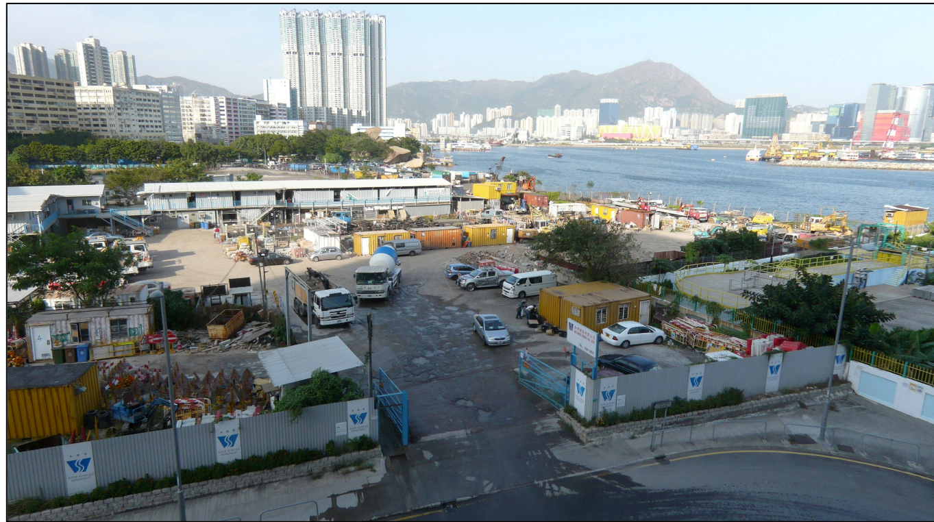
Existing View from South – A.B.P. Centre
