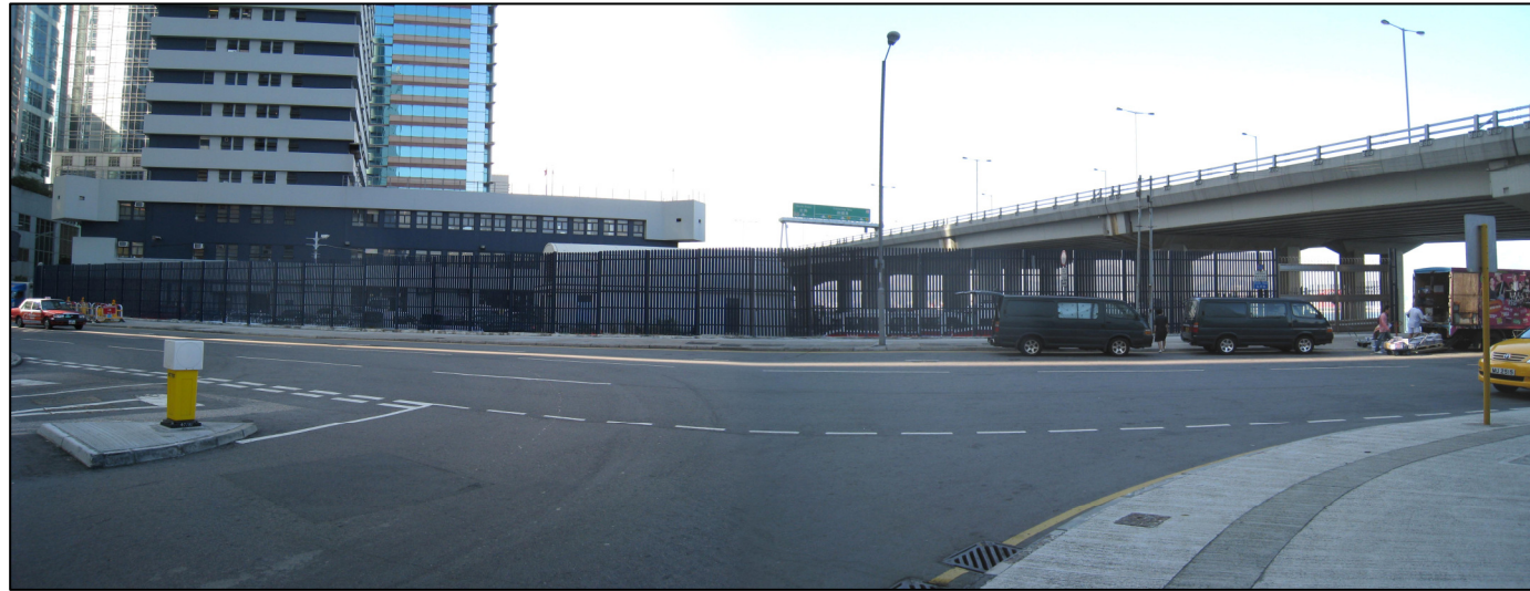
Existing View from Southeast – Hoi Chak Street
