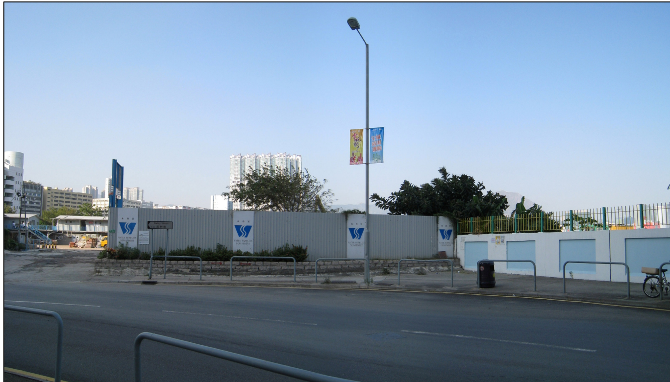
Existing View from South – Bailey Street
