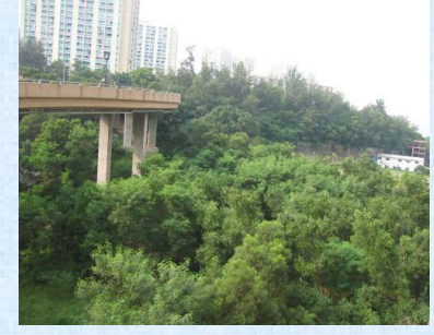
LR5 – Trees on slope along Tsing Yi Road
