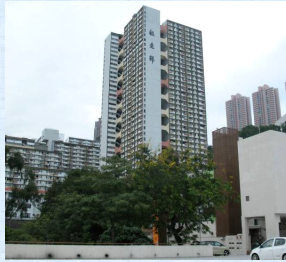
VSR1 – Ha Kwai Chung Residential Area
