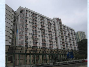
VSR15 – Tsing Yi Residential Area
