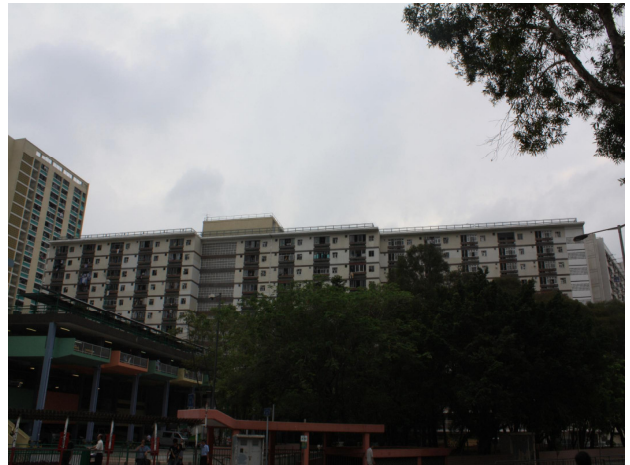
Cheung Ching Estate - Ching Kwai House (CKH)
