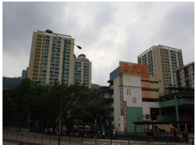
Cheung Ching Estate - Ching Wai House (CWH, right) Cheung Ching Estate - Ching Yung House (CYH, left)
