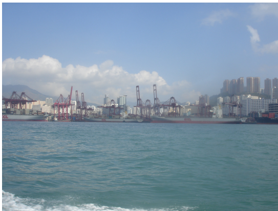
Plate 11. A section of the container terminal that was surveyed as part of this project.
