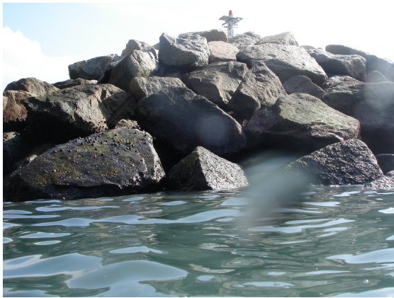
Plate 2. The quarry rock protection mound immediately out from T2.
