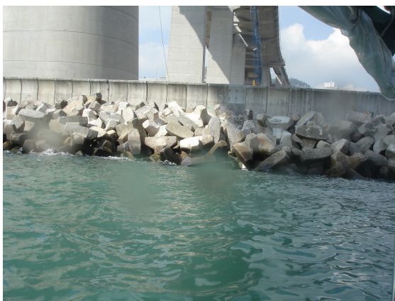
Plate 12. A dolos seawall. This wall seemed new in that there was very little settled on it.
