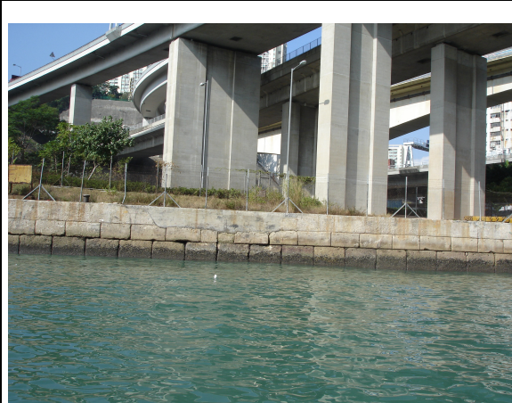
Plate 1. The seawall at T2.
