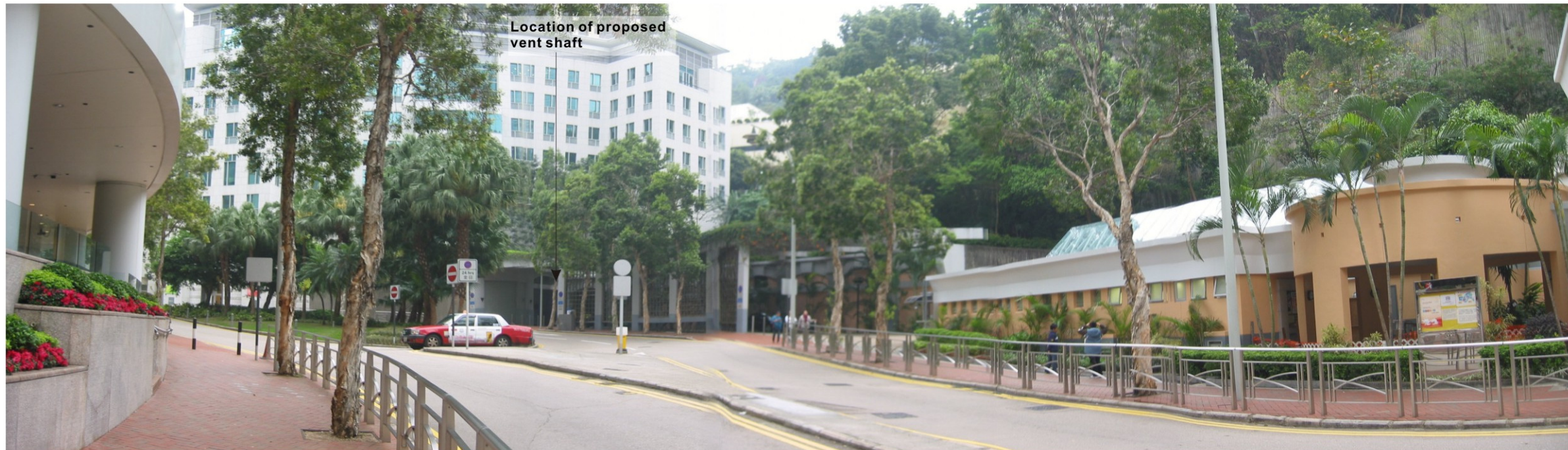
Existing Condition Vantage Point C - View south at Supreme Court Road in front of Hong Kong Park entrance looking towards the proposed vent shaft.
