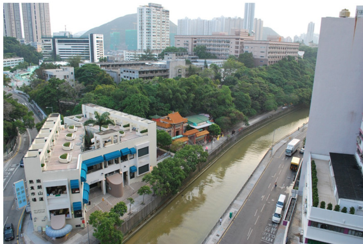
Existing Condition Vantage Point H - View west at an elevated level of industrial building at Heung Yip Street looking towards the proposed viaduct from WCH Station
