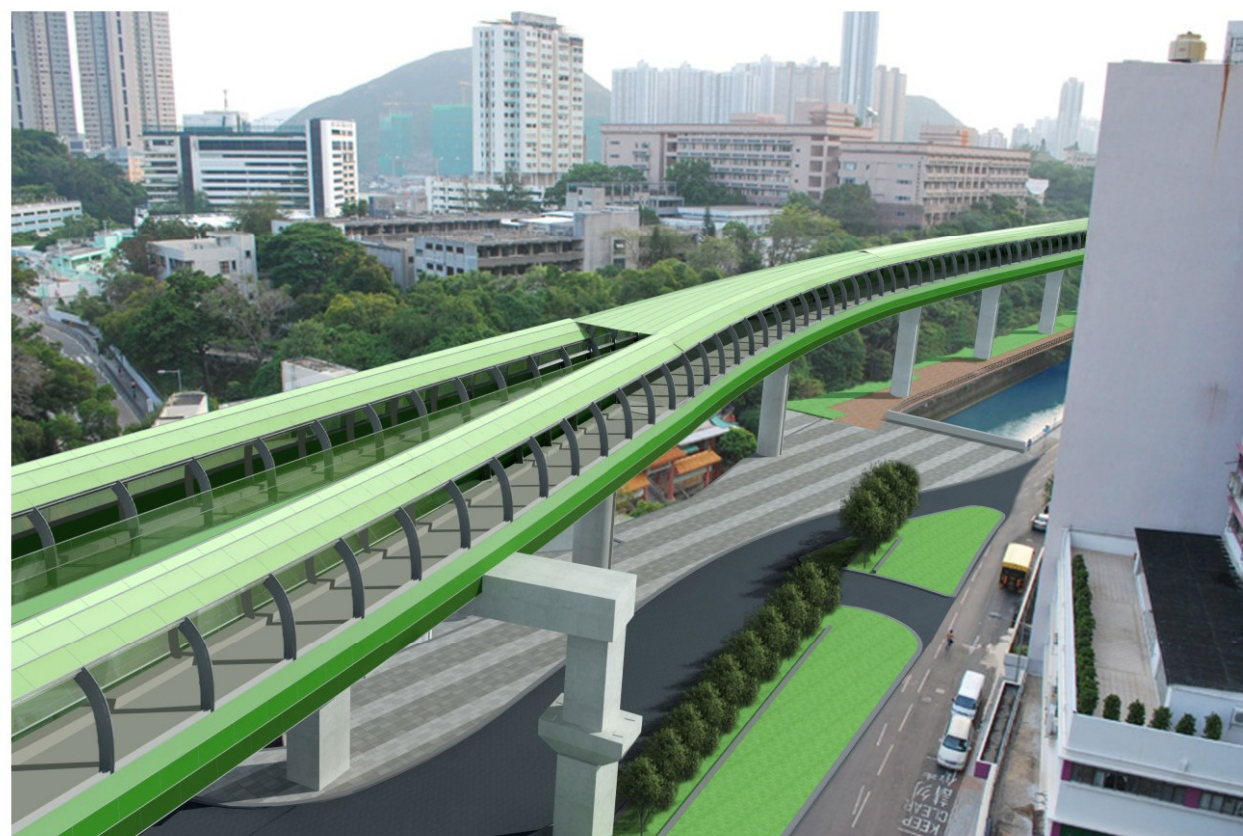
Year 10 of Operation Phase with landscape mitigation measures fully established
