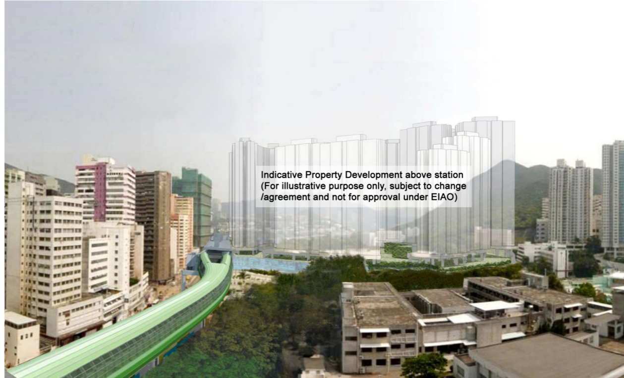
Year 10 of Operation Phase with landscape mitigation measures fully established
