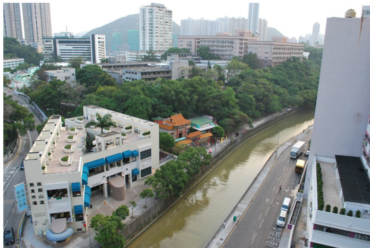
Existing Condition Vantage Point H - View west at an elevated level of industrial building at Heung Yip Street looking towards the proposed viaduct from WCH Station
