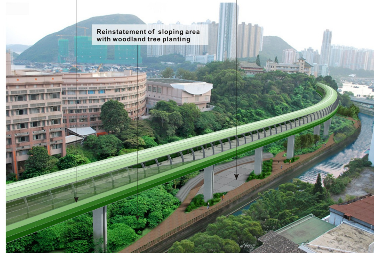
Viaduct with partially enclosed noise barrier designed and colourful curvy panel to disguise the engineered form of the viaduct
