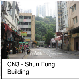
CN3 - Shun Fung Building
