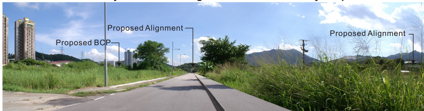
View Towards the Project without Mitigation Measures on Day 1 Operation from VP3
