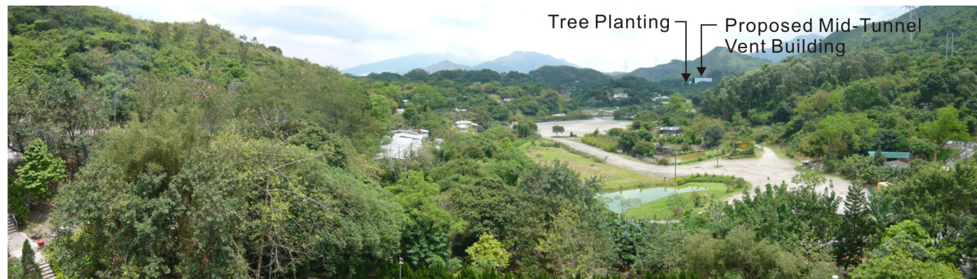
View Towards the Project with Mitigation Measures at Year 10 Operation from VP9
