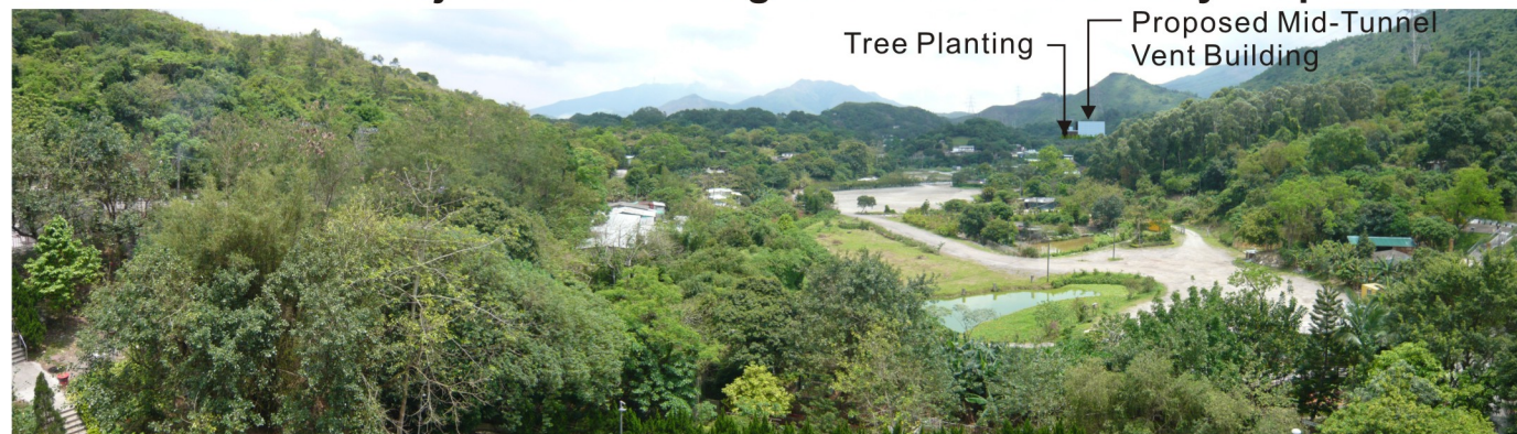
View Towards the Project with Mitigation Measures on Day 1 Operation from VP9
