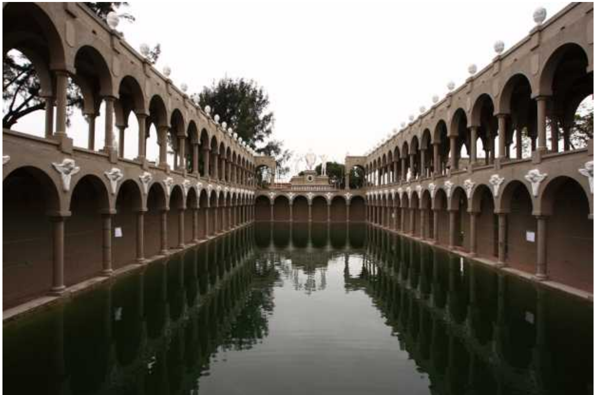
The Courtyard, used as a Water Storage Facility
