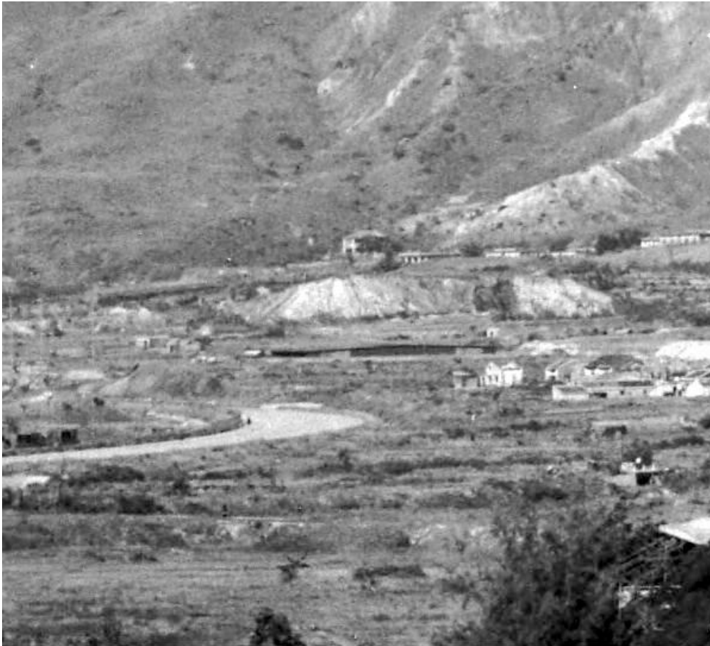
Plate 2: View to west across Tai Hom landscape in early 1950s showing the landscape before the squatter settlement and roof of the RAF hangar in mid photo.
