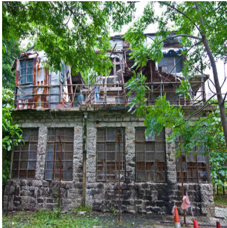
Photograph 2 Stone House, No. 4 Tai Koon Yuen
