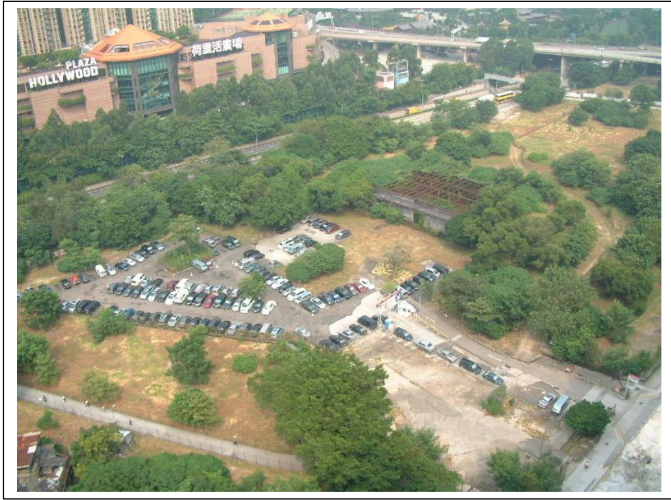
Plate 1.3 Aerial view of disused Former Royal Airforce Hangar in poor condition (circa 2007)
