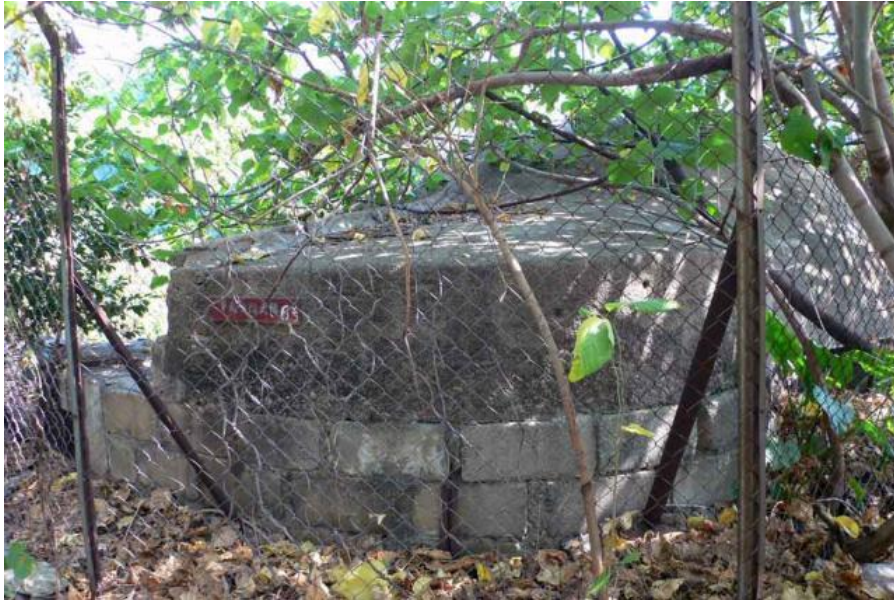
Plate 1.5 A fortified old pillbox at the Tai Hom area
