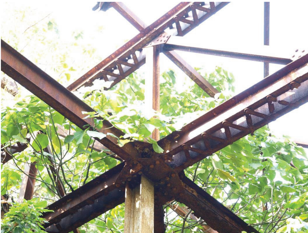
Photo P1070437 – Location 06 – roof structure and support
