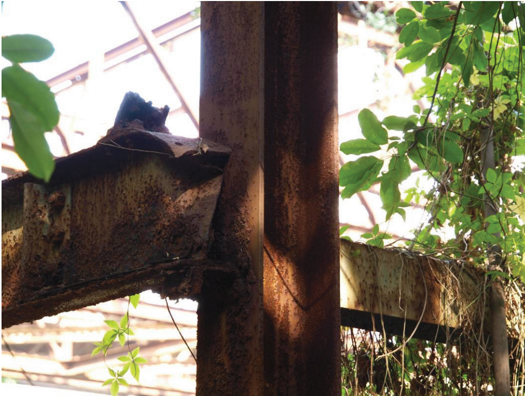
Photo P1070541 – Location 21 – at mid height of column
