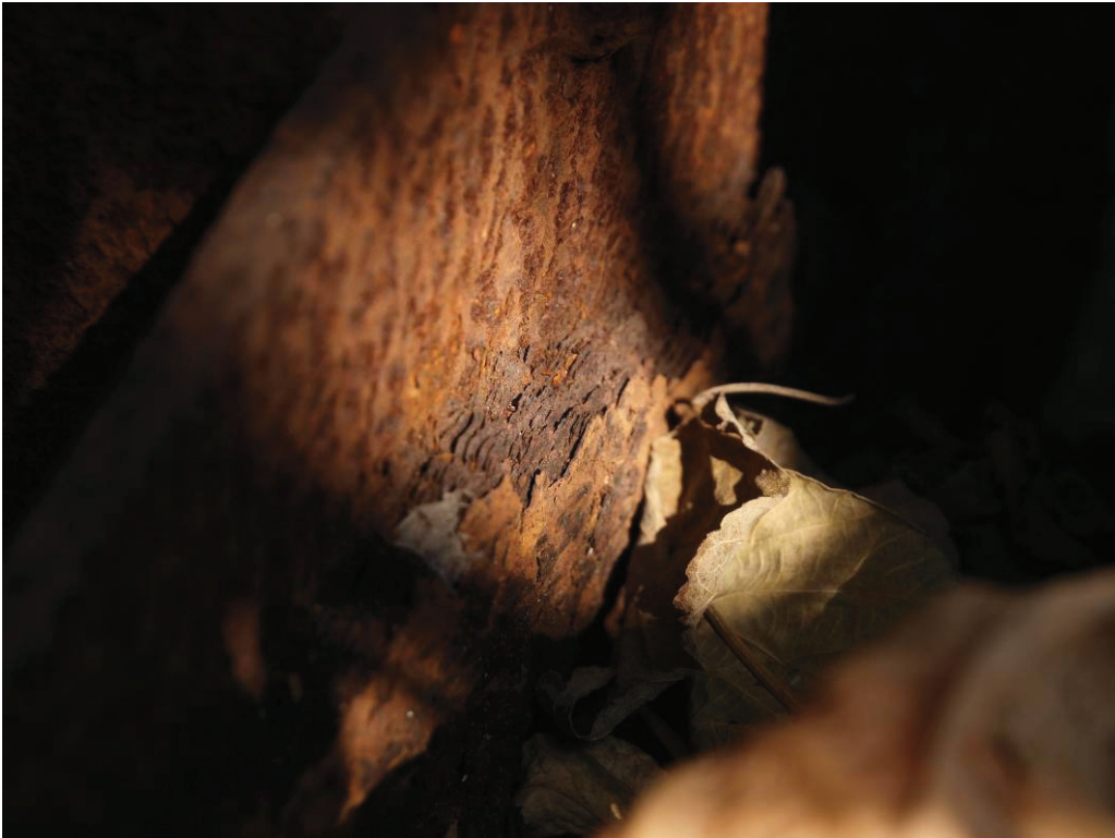
Photo P1070647 – Location 31 – roof structure
