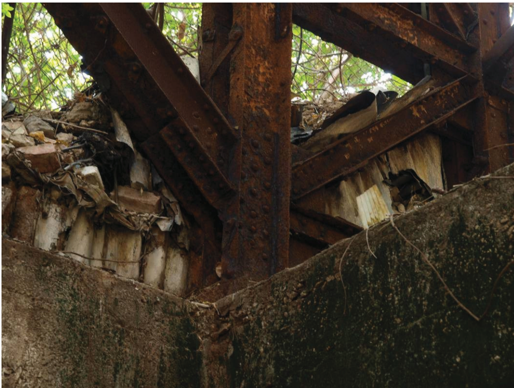
Photo P1070591 – Location 29 – roof structure and support
