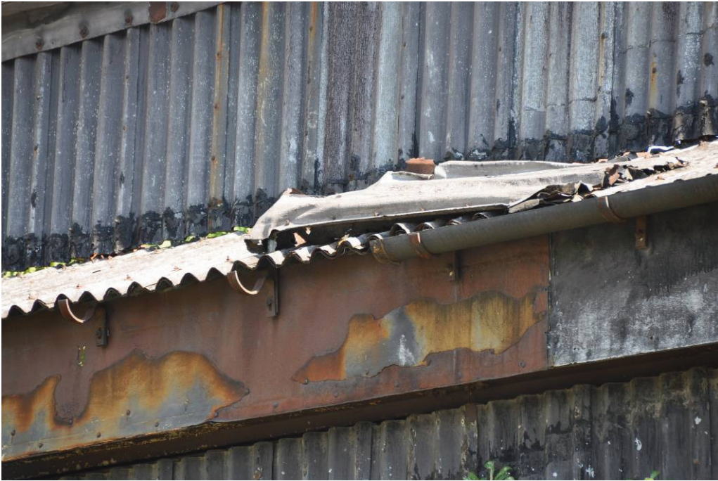
Photo DSC_0642 – Front of structure – typical cladding detail
