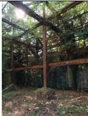
Photo 1 – Steel-I-column with concrete footing
