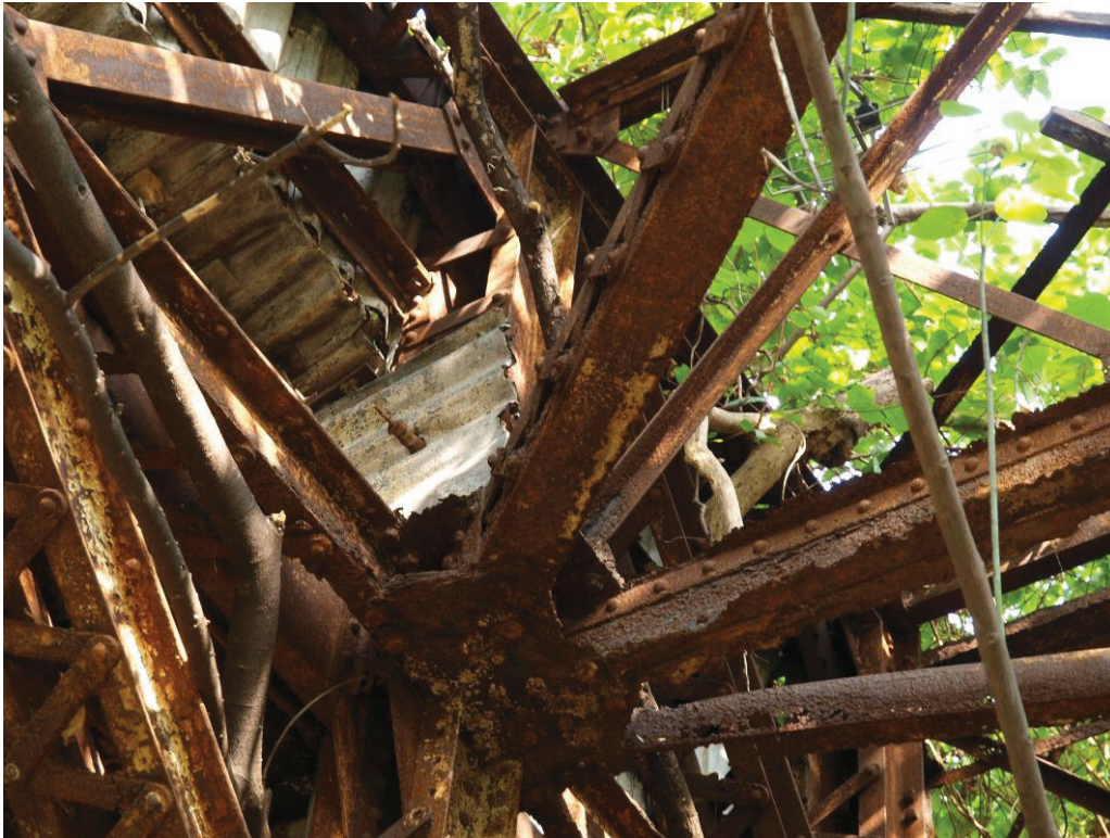
Photo P1070434 – Location 04 – roof structure
