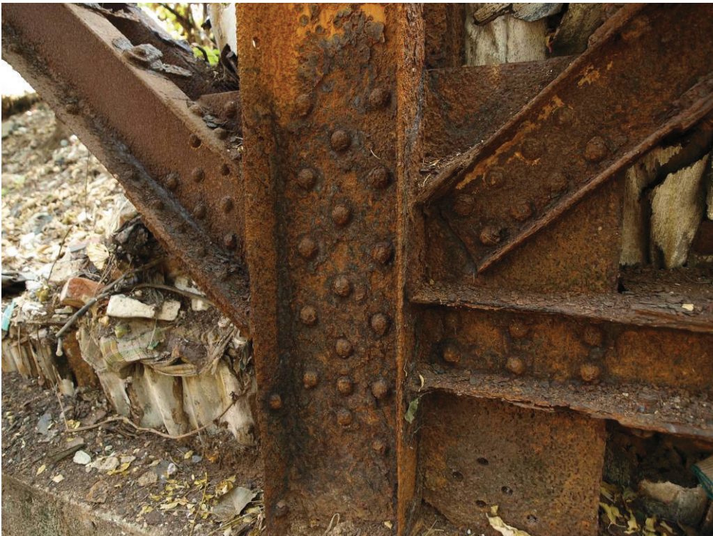
Photo P1070631 – Location 31 – roof structure and support
