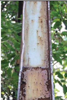
Photo 7 – Buckle at I-beam
