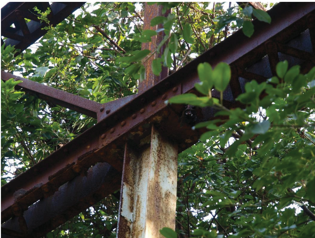
Photo P1070575 – Location 26 – roof structure and support
