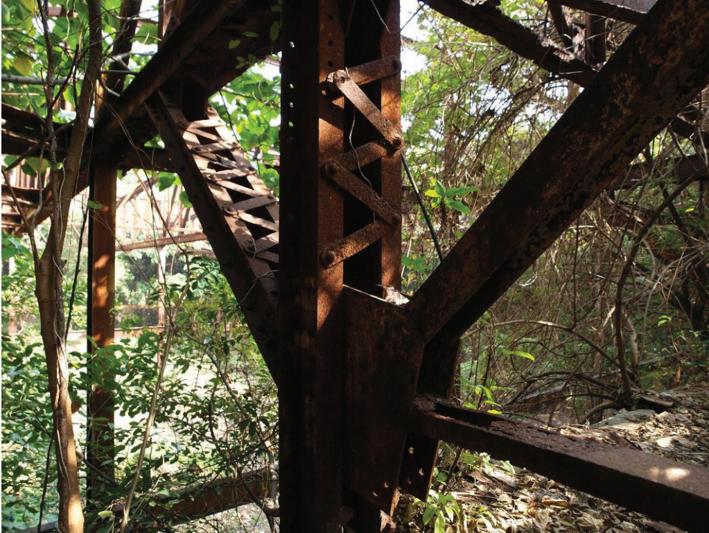
Photo P1070613 – Location 31 – roof structure
