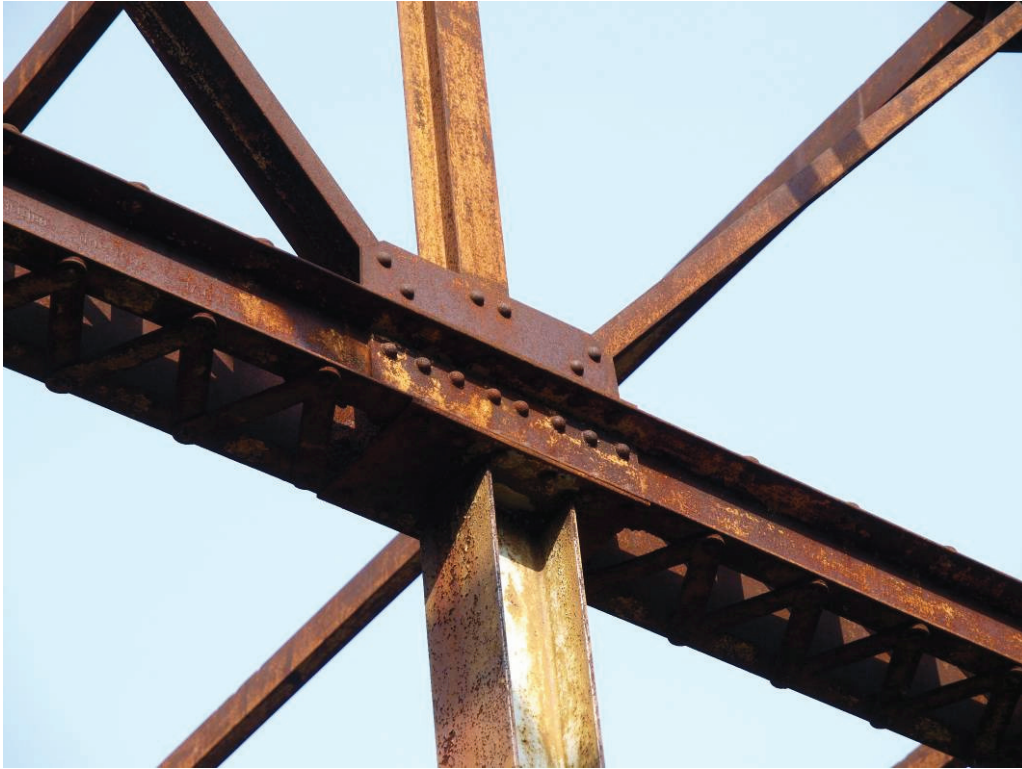
Photo P1070477 – Location 12 – roof structure and support
