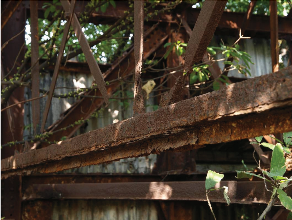
Photo P1070648 – Location 31 – roof structure
