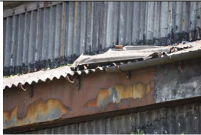
Photo 5– Corrugated zinc sheet with waterproofing bitumen sheet coating
