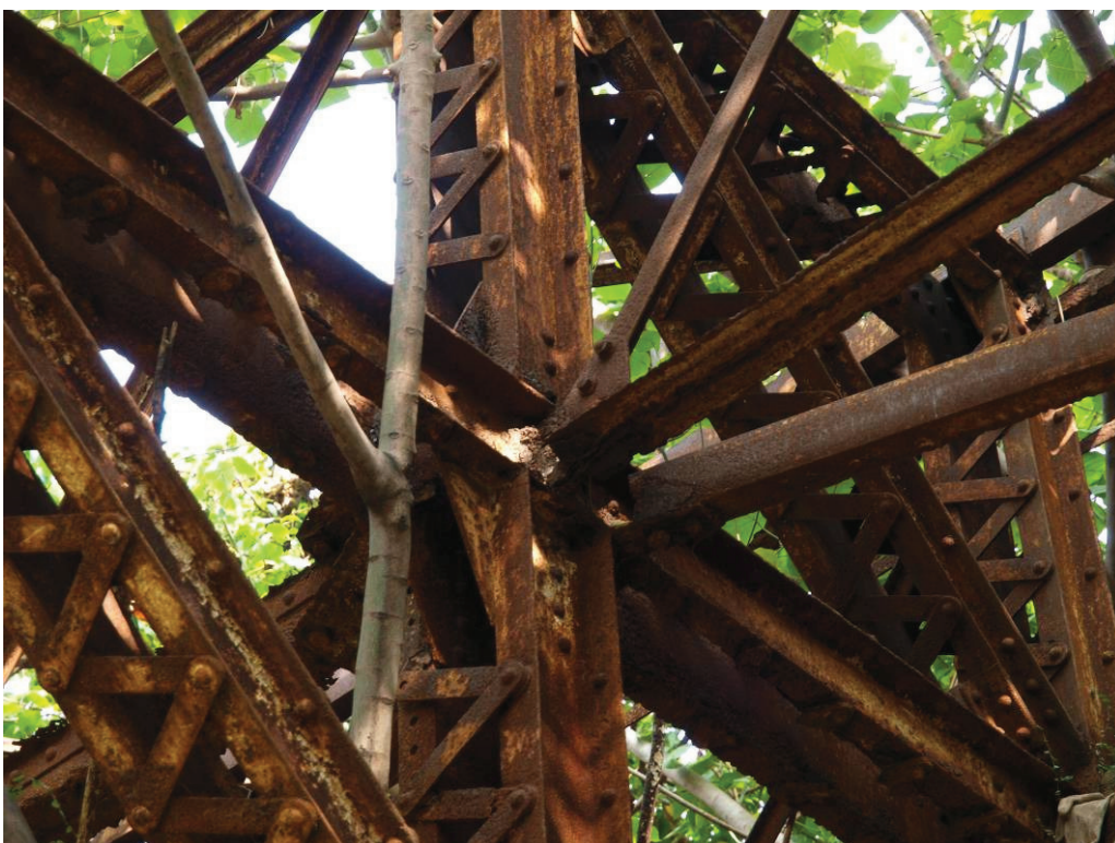
Photo P1070460 – Location 9 – roof structure
