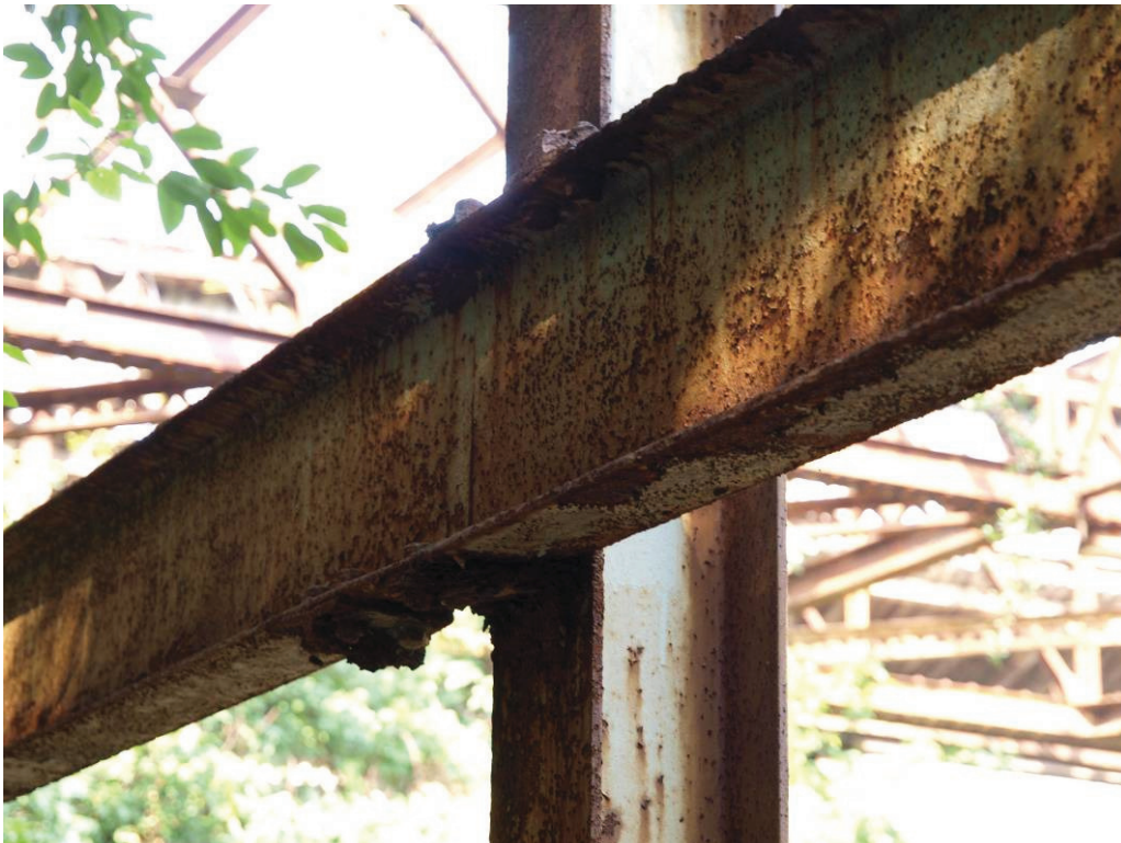
Photo P1070508 – Location 16 – at mid height of column
