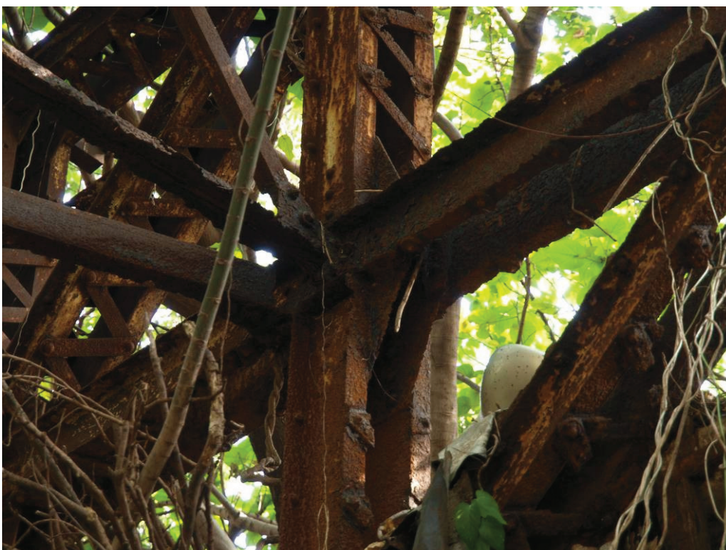
Photo P1070596 – Location 30 – roof structure
