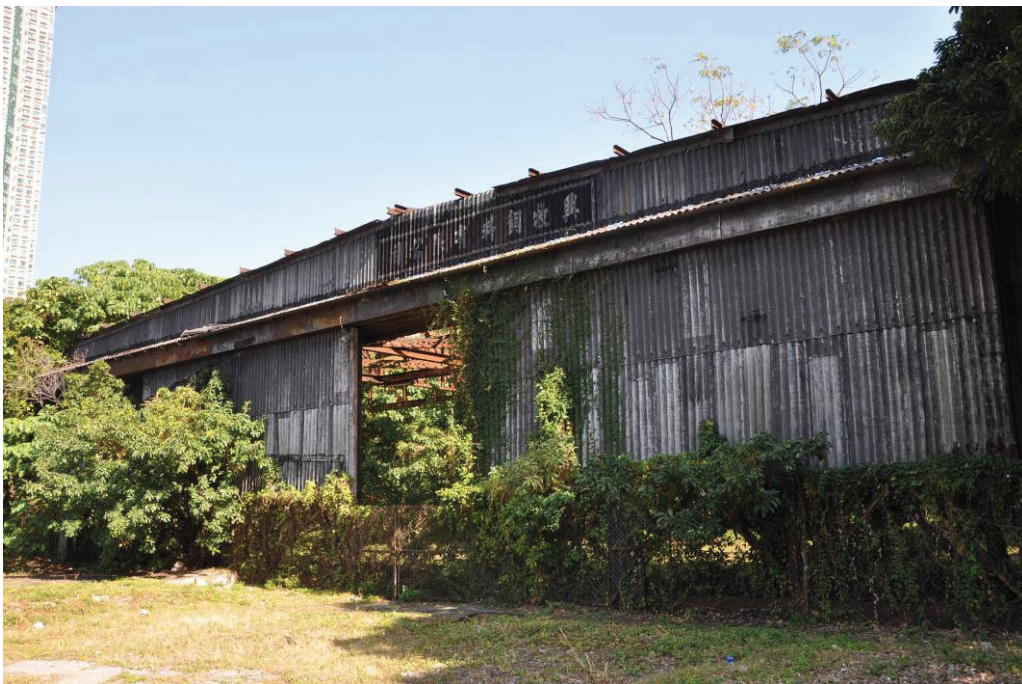
Photo DSC_0628 – Front of structure
