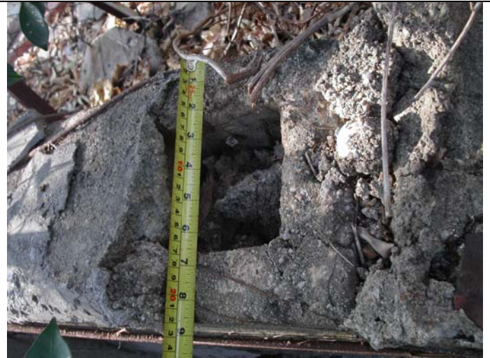
Photo 25 – Hollow Masonry Unit
