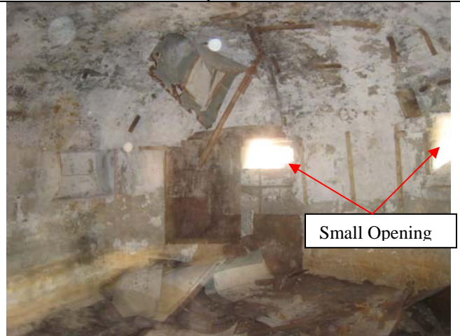
Photo 28 – Internal of Pill Box
