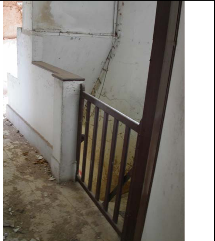
Photo 21 – Wooden Gate at 1/F of staircase
