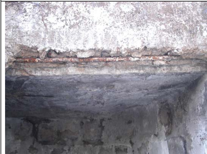
Photo 26 – Reinforcement Concrete Roof Slab
