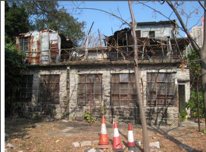
Photo 18 – Steel Frame Window
