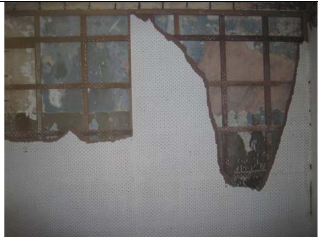
Photo 12 – Timber Frame Partition
