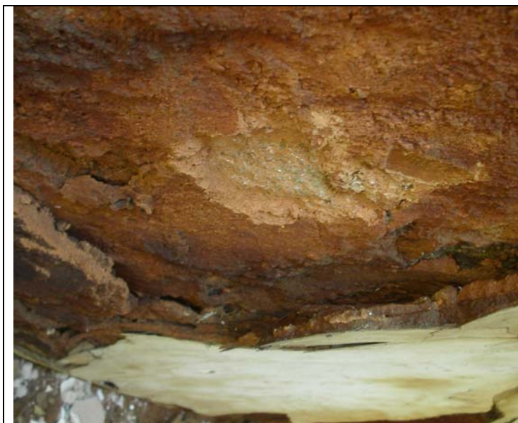
Photo 3 – Chunam Mortar & Cement Sand Plaster
