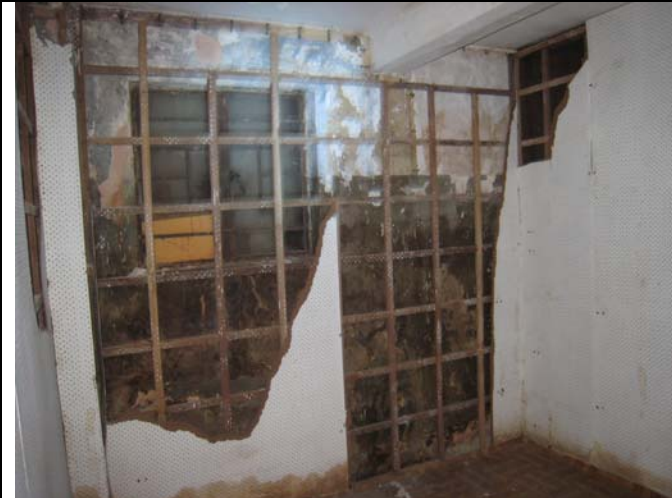
Photo 20 – Audio Room for Film Production at G/F
