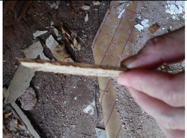
Photo 10 – 2 ~ 3 mm thick of cement sand plaster
