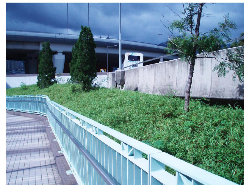
HUH/LR3.5 - ROADSIDE AMENITY AREAS AT SALISBURY ROAD AND HONG CHONG ROAD ABOVE THE PORTAL OF CROSS HARBOUR TUNNEL
