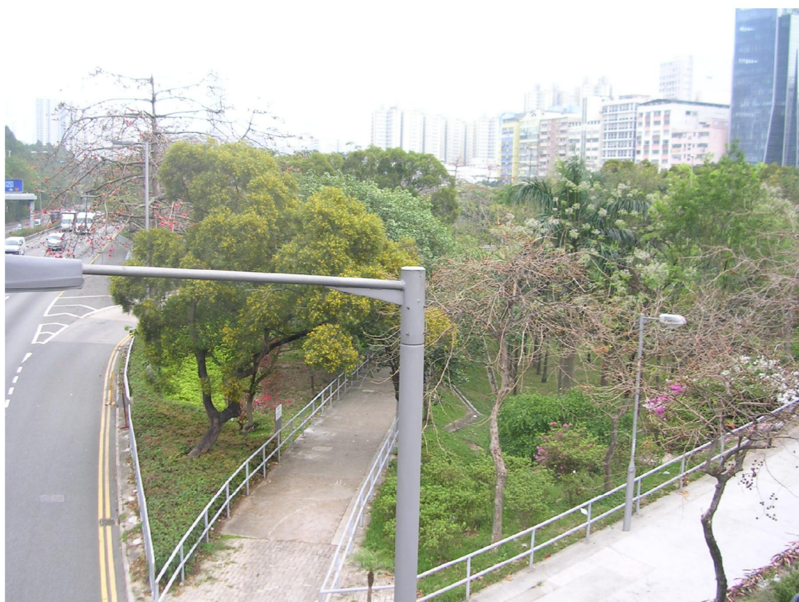
DIH & KAT - LR 3.2 - AMENITY AREAS AT JUNCTION OF LUNG CHEUNG ROAD AND PO KONG VILLAGE ROAD
