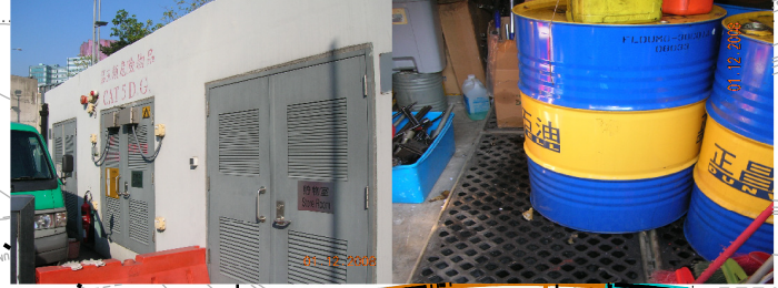
DANGEROUS GOODS AND CHEMICAL STORAGE ROOM OF THE INTERNATIONAL MAIL CENTRE
