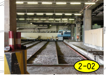
INTERCITY LOCOMOTIVE TRAVERSER (APPROXIMATELY 800 m 2 ) AT HUNG HOM FREIGHT TERMINAL
