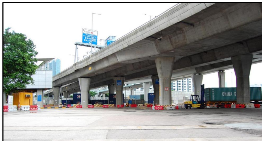
OU2 FREIGHT TERMINAL
