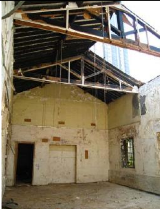
The original roof structure of Laboratory Block, Old Victoria Barracks
