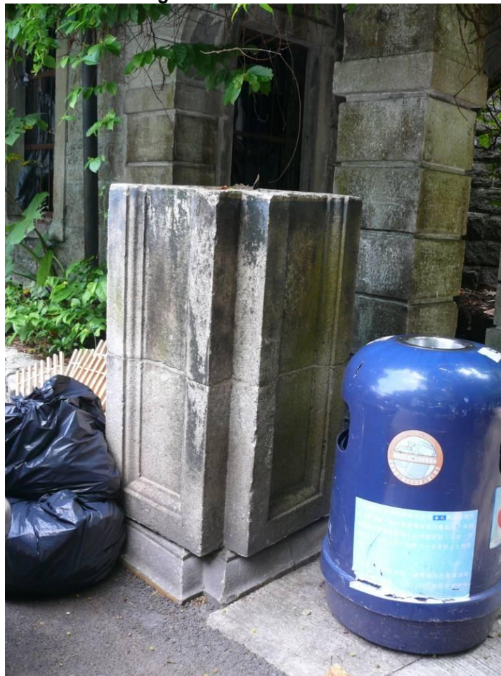
Upper portion of one of the Pier is missing
