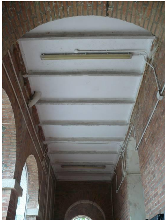
Steel beams of first floor of North Wing , Old British Military Hospital
