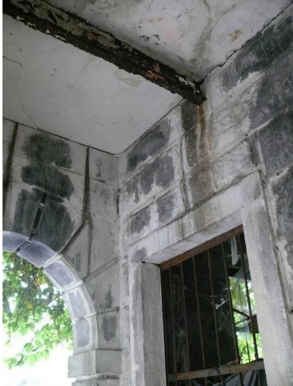
Arch structure and iron beam of ceiling of Guard House, Old British Military Hospital
