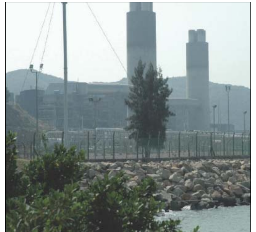
VSR6 - BLACK POINT POWER STATION
