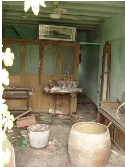
Interior View of No. 63 Cheung Uk
