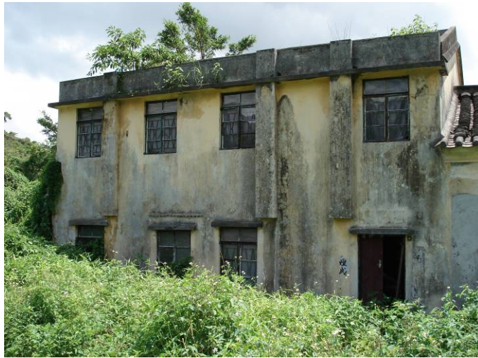
Rear View of No. 62 and 63 Cheung Uk
