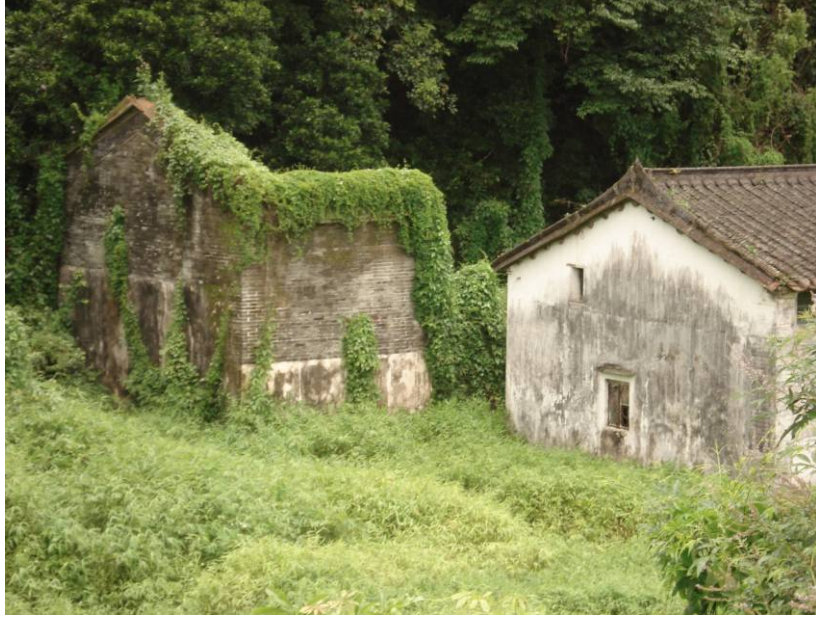
General View of Ruined Village House
