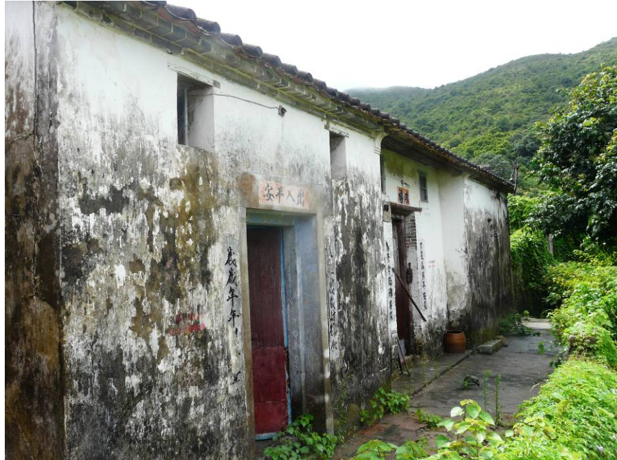
General Front View of No. 43
