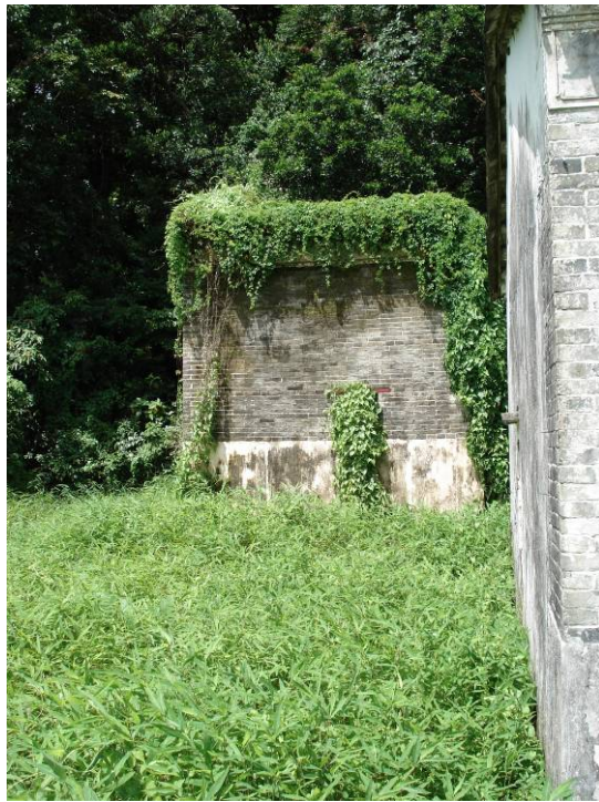
Front View of Ruined Village House
