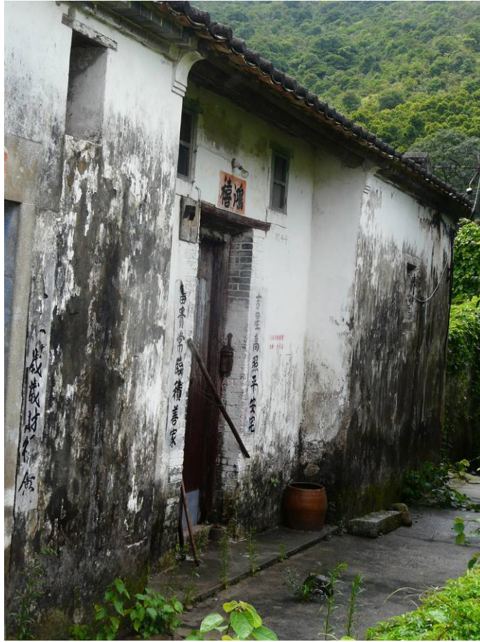
General View of No. 44
