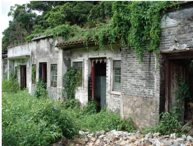
Side View of No. 13 Cheung Uk
