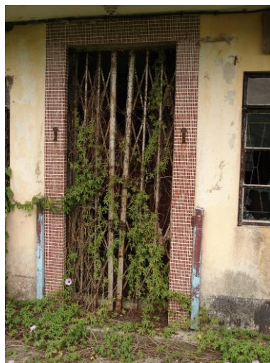
Entrance Door and Gate of No. 62 Cheung Uk
