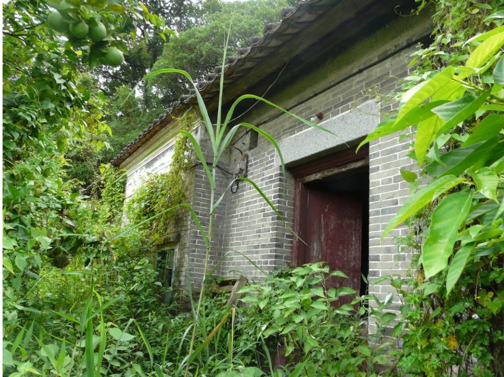
Front view of Nos. 15 and 16 Cheung Uk
