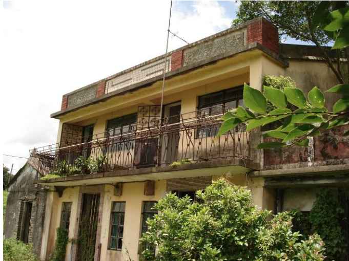
General View of Nos. 62 and 63 Cheung Uk
