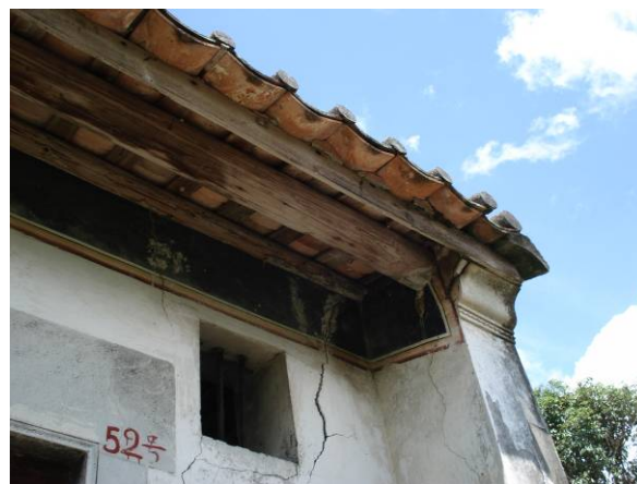
Tiled Roof and Beams
