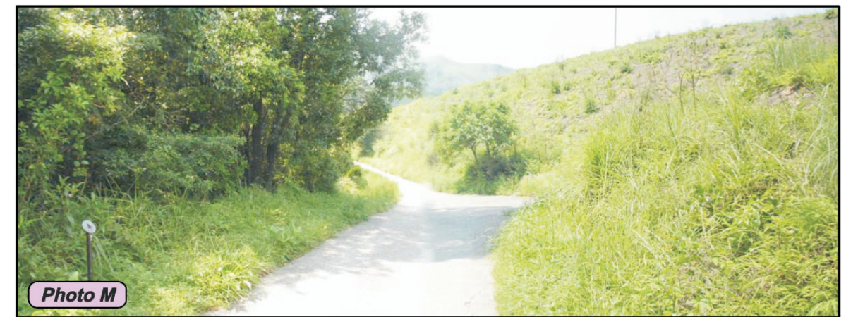
Existing Road Condition at Section 8 - 8
