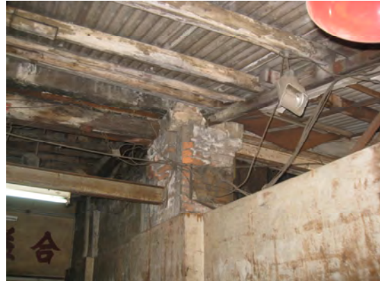
Example of a brick support structure in a unit on Waterloo Road
