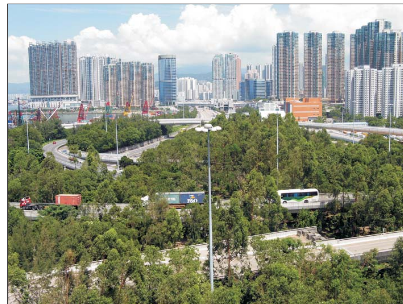
T1.1 West Kowloon Highway
