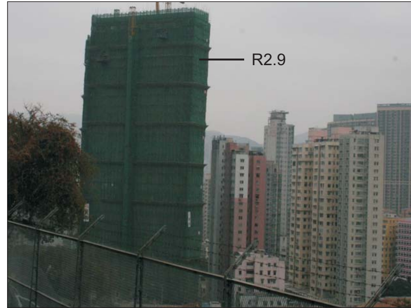
R2.9 Hong Kong Polytechnic Student Hostel Development
