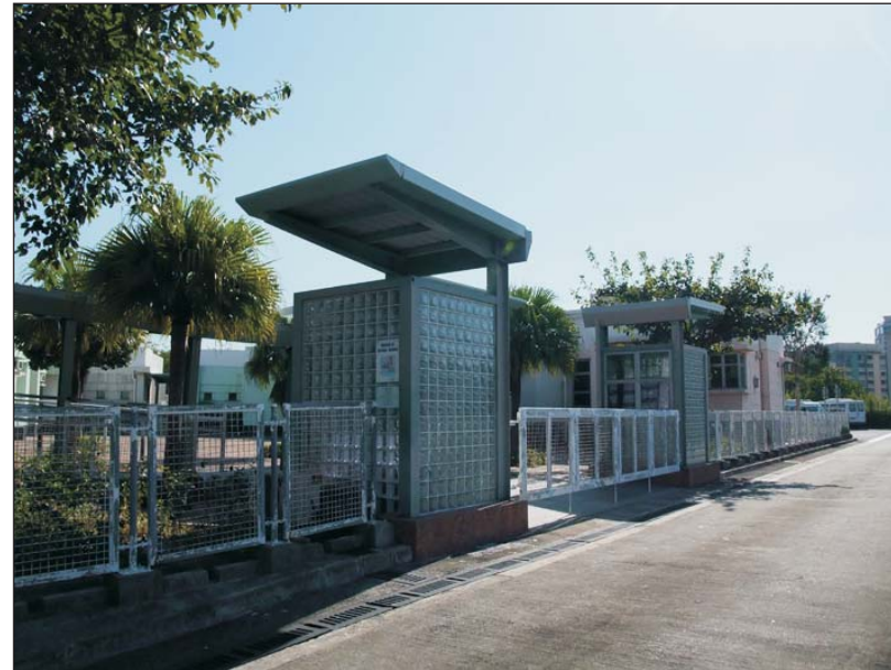
GIC2.4 Housing Authority Mock-up Centre
