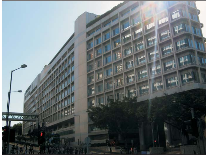
GIC2.3 Housing Authority Headquarters
