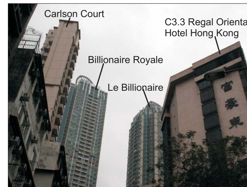
R3.5 High Rise Developments along Prince Edward Road East
