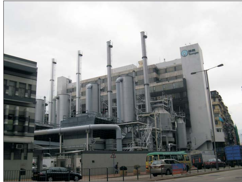
O3.1 The Hong Kong and China Gas Company Limited Ma Tau Kok Control Centre
