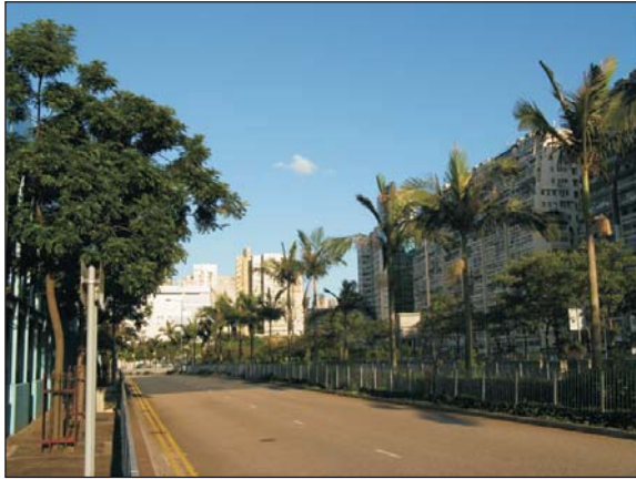
LR1.3b Roadside Planting along Hoi Wang Road, Area Yan Cheung Road and Ferry Street Area
