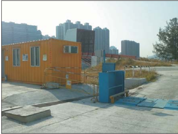
LR1.5c Disturbed Area at Kwai Chung
