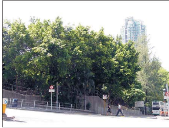
LR2.4a Vegetation on Man-made Slopes along Chung Hau Street and Fat Kwong Street
