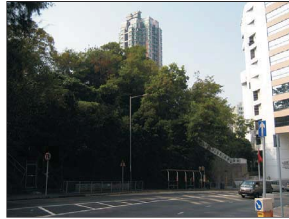
LR2.4a Vegetation on Man-made Slopes along Chung Hau Street and Fat Kwong Street
