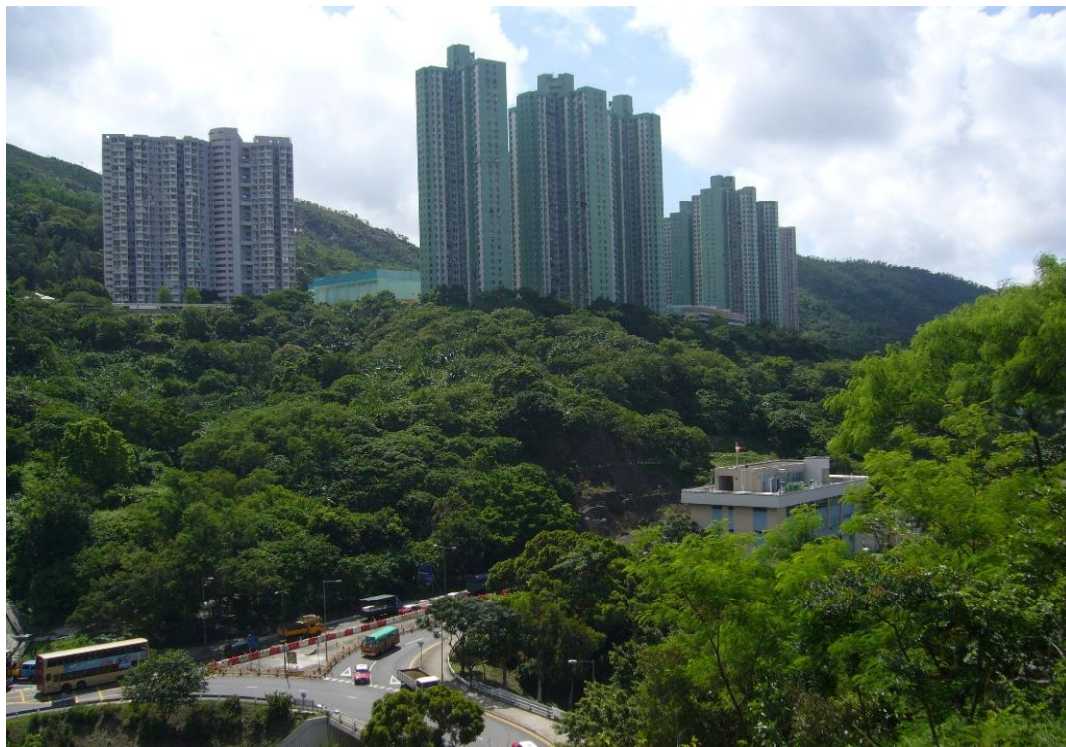
Disturbed Woodland between Kwong Tin Estate and Lei Yue Mun Road
